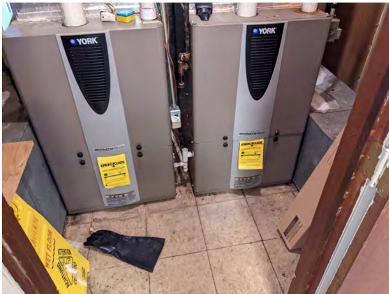
Forced air furnaces in mechanical room.
