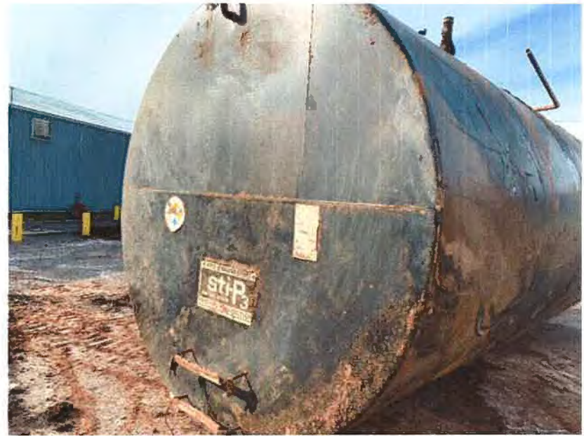
View of 15,000-gallon Diesel Fuel Tank
