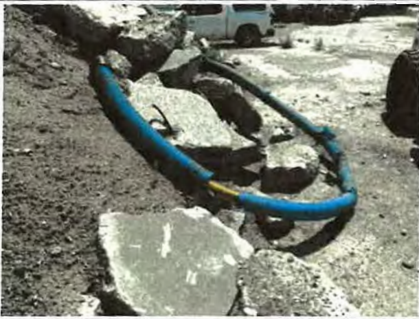
Removed vent and fill piping
