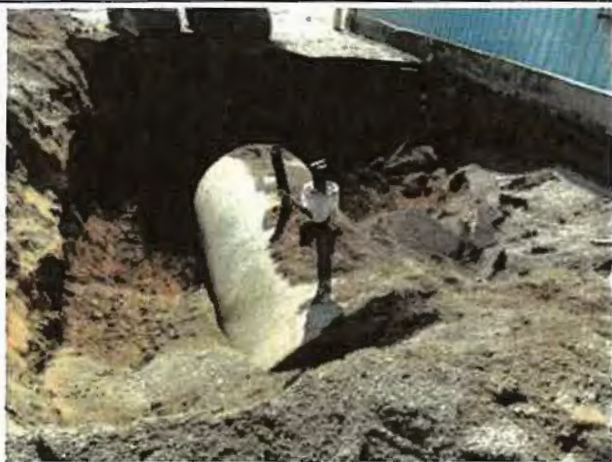
4,000-gallon waste oil UST during excavation
