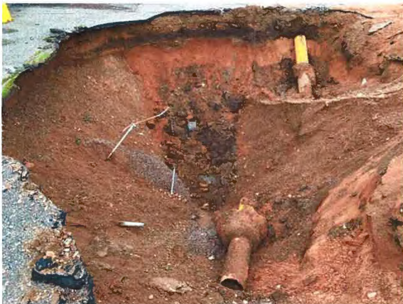
Gasoline UST tank excavation
