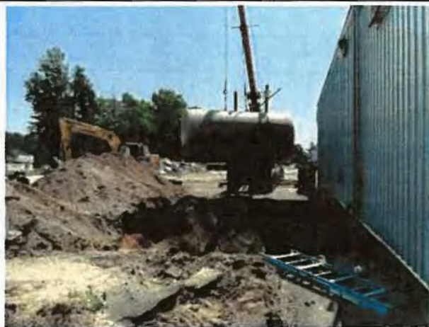
4,000-gallon waste oil UST being removed from excavation
