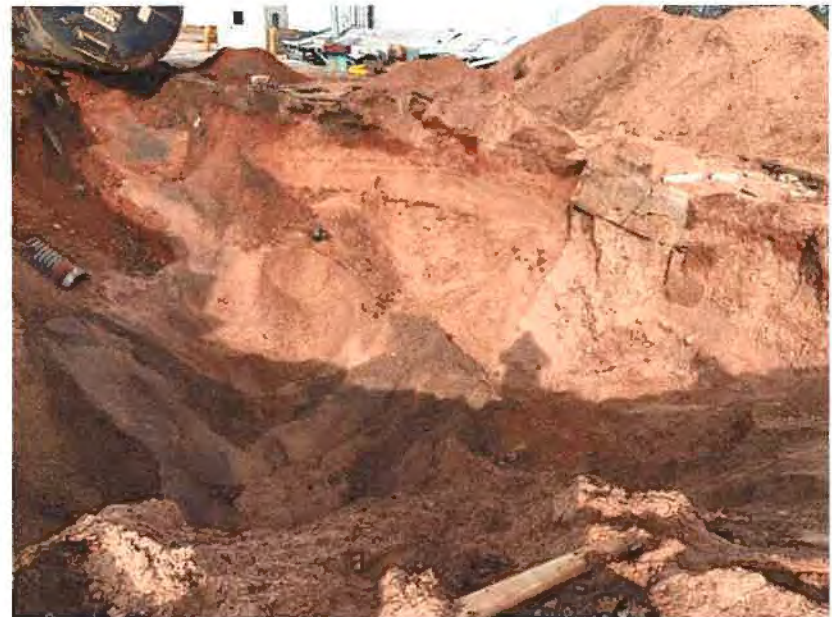
Diesel Fuel UST tank excavation
